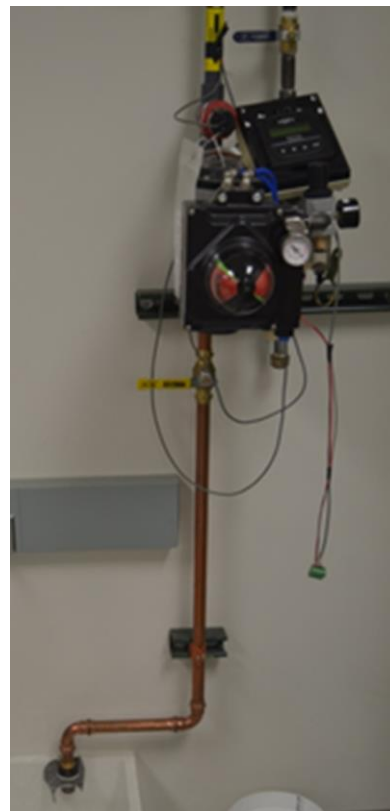
Fig. 6 Abandoned Flow Control Valve
