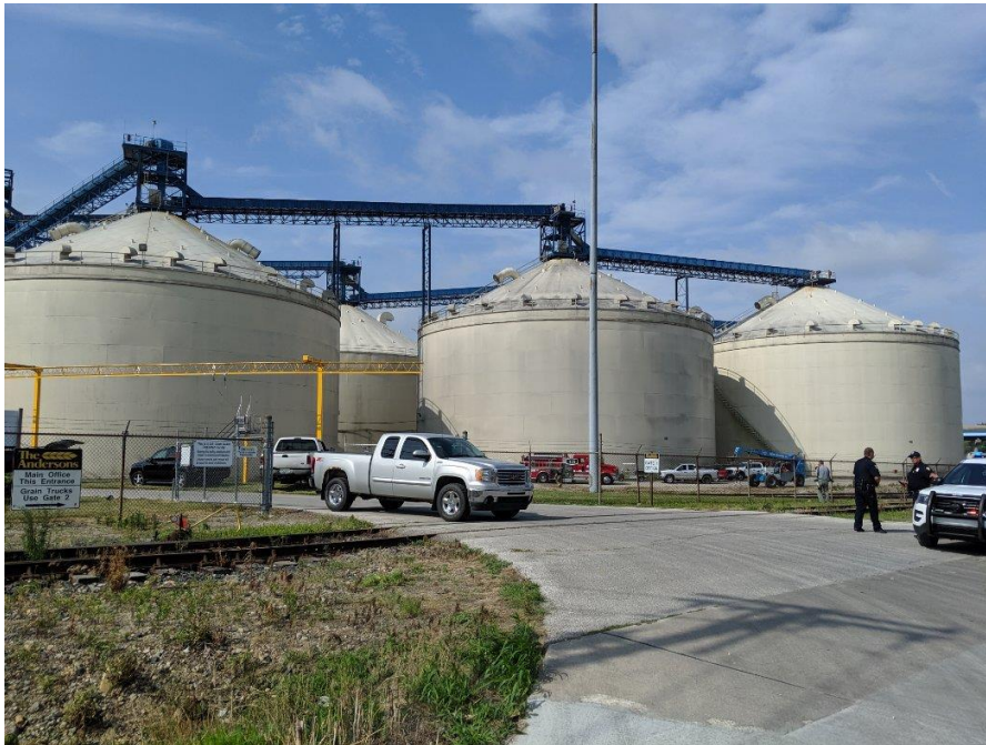
Fig. 10-8 Andersons Grain Handling Facility
