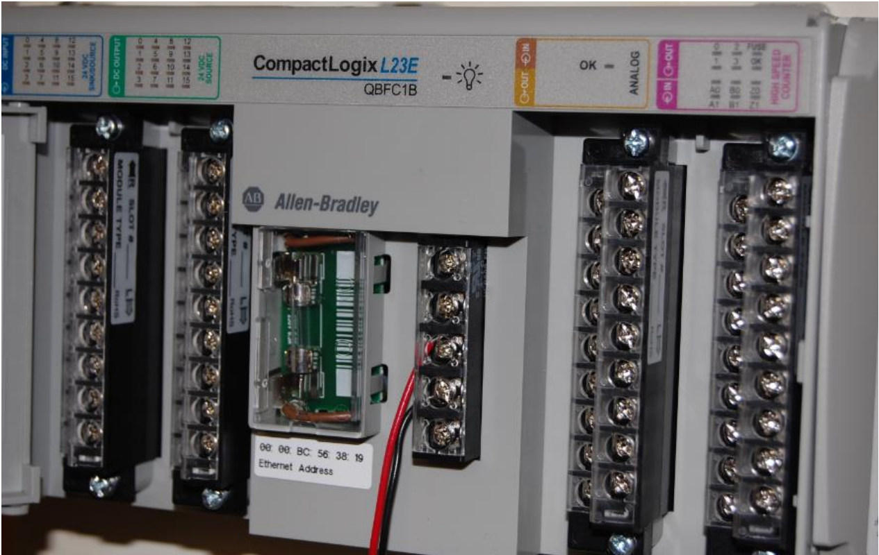
Fig. 3-19 View of CompactLogix L23E with Wiring Exposed
