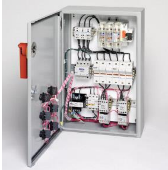
Fig. 9-33 Industrial Control Panel with High SCCR Rating
